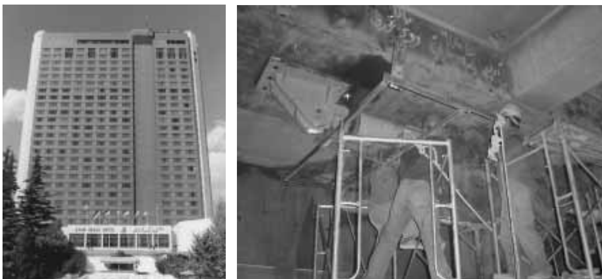
Figure 10. Application of hydraulic dampers as a part of the retrofitting plan for a tall hotel building in Tehran.
