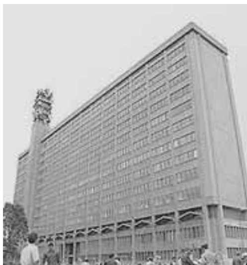
Figure 5. Telecommunication building in the central part of Tehran built in early 1970's. Two Teflon plates with rubber in between are installed between the basement and the ground floor columns of the building.
