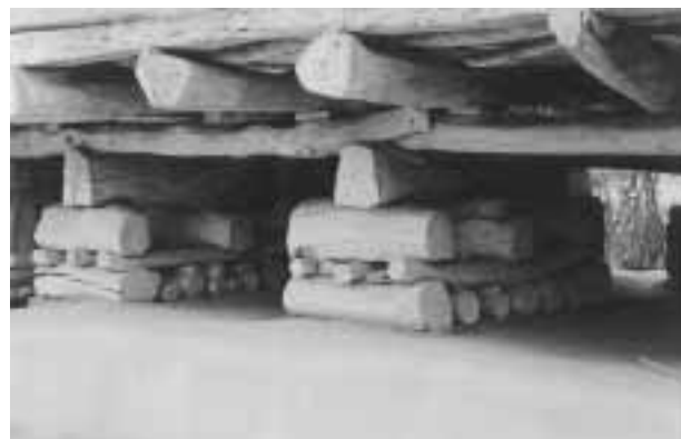
Figure 4. Use of pieces of wood between the ground and the bearing walls of traditional houses in Lahijan, north of Iran. This demonstrates a base isolation technique that was applied long before the introduction of modern base isolation technology.
