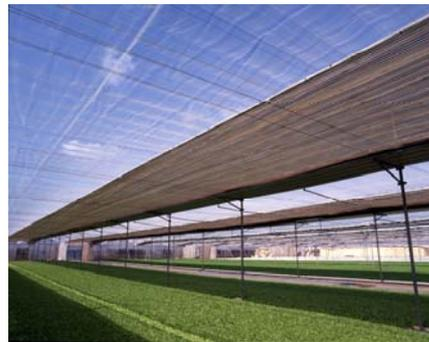
The shading screens are made up by aluminium and acryl. It can be placed inside or outside the greenhouse. This kind of screen can get a temperature drop up to 10 °C because it lets the air flow and, at the same time, this screen shades the greenhouse.
