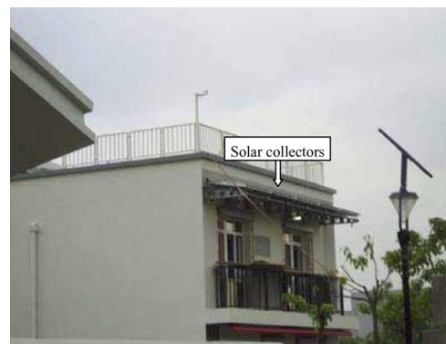
Fig. 7. A picture showing use of collector in the sunshade [5]
